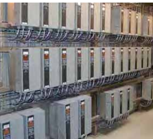
A typical drive installation with multiple frequency converters all installed on the same power supply often requires supplementary harmonic mitigation to avoid harmonic voltage distortion.
